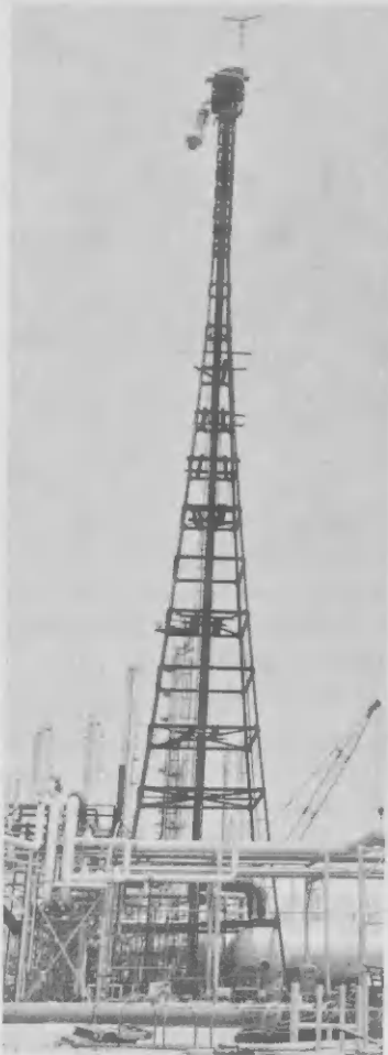
At left, the tip is shown dangling near the 250-ft. high Alky II stack. At right, the tip reaches its destination.
